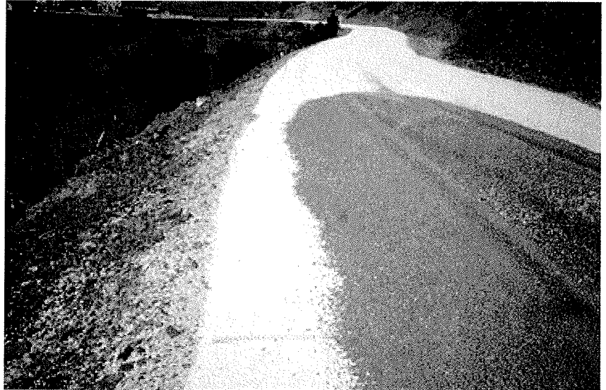
These two photos depict a the good job of spreading done by a county highway department using tandem end-dump trucks. The skill of the drivers makes this job look easy. Notice also the grader is ready to begin processing the material.
