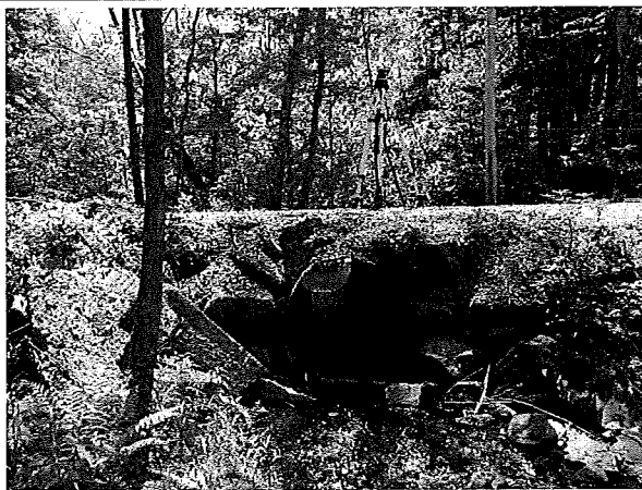
Photo 1: Inlet of the 48" culvert under Rogers Road.
