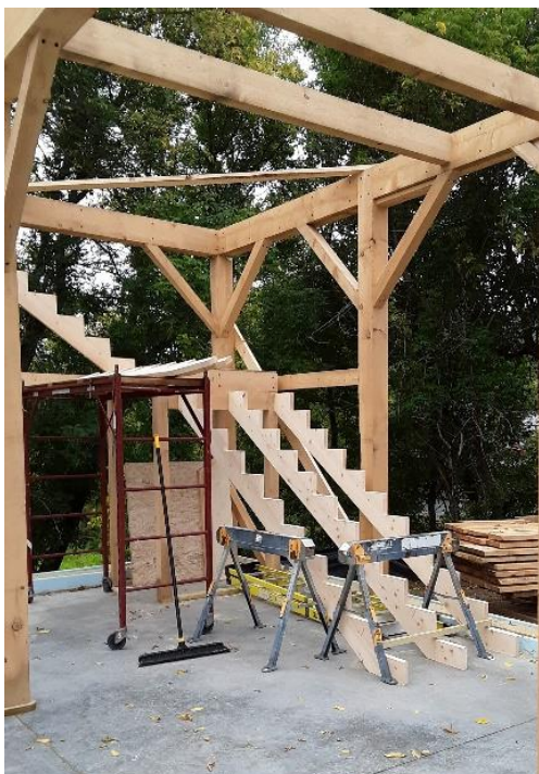
Construction of staircase to second floor
