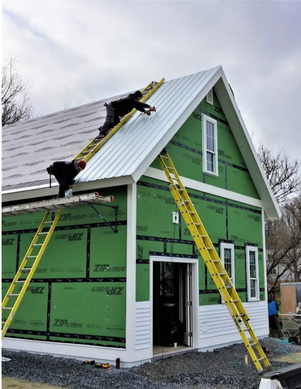
Roof and siding installation.
