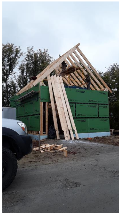
Adding the trusses!
