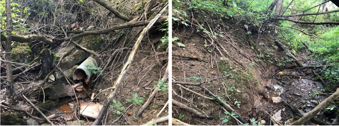
Outlet of 18" culvert in poor condition (left) and erosion in swale to Browns River (right)
