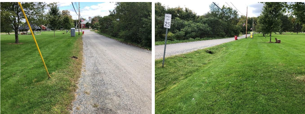
Looking east at elevated grass shoulder along Common Road (left) and looking west at 18" culvert inlet beneath Common Road, the potential location for a stormwater retrofit practice (right).
