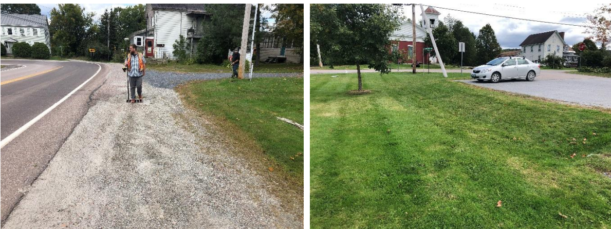
Catch basin along Route 128 (left) and grassed swale that could receive redirected runoff (right)
