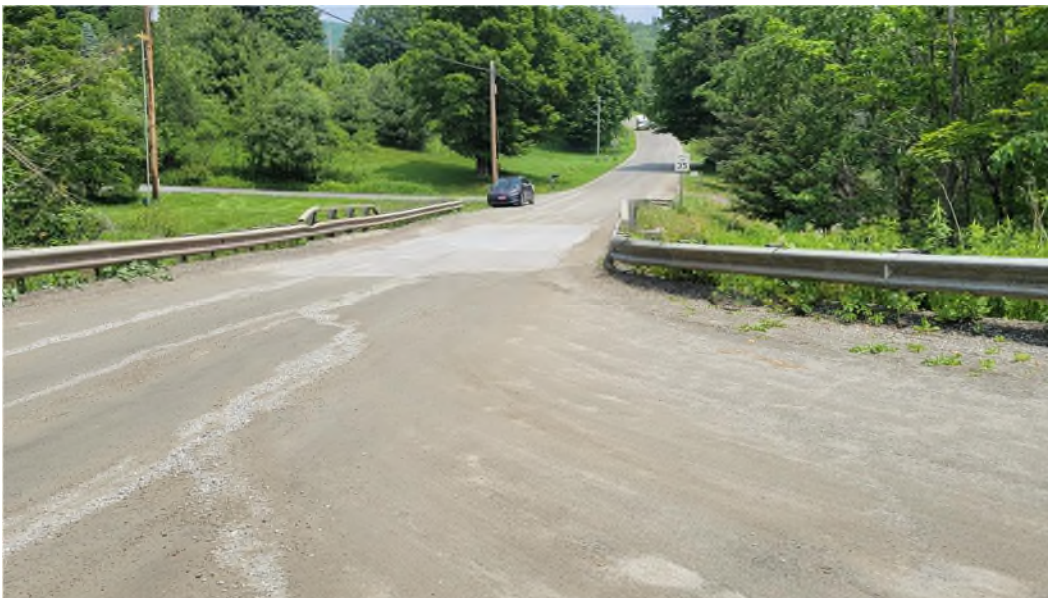
Figure 4: Looking north, towards right, from Maple Tree Lane
