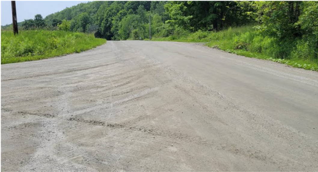
Figure 5: Looking south, towards left, from Maple Tree Lane
