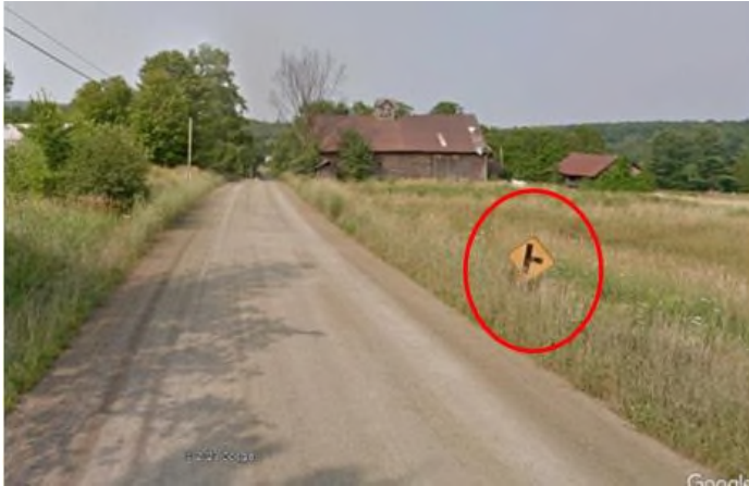
Figure 9: Existing Intersection Warning Sign
