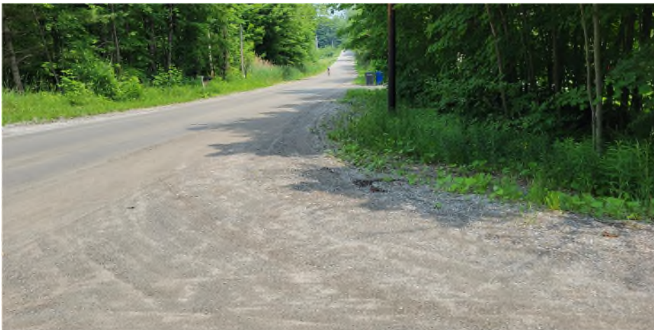
Figure 2: Looking north, towards right, from Phelps Road
