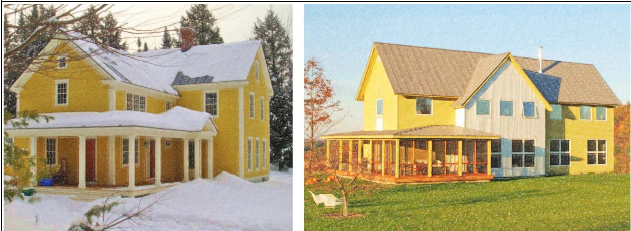
THE NEW HOUSE (LEFT) CLOSELY REPLICATES THE DESIGN OF A HISTORIC VERMONT FARMHOUSE. THE NEW HOUSE (RIGHT) IS A CONTEMPORARY INTERPRETATION OF THE VERMONT VERNACULAR. THE BUILDINGS ARE SIMILAR IN SCALE. THEY SHARE FEATURES LIKE ROOF FORM, CROSS-GABLES AND THE PORCH.
