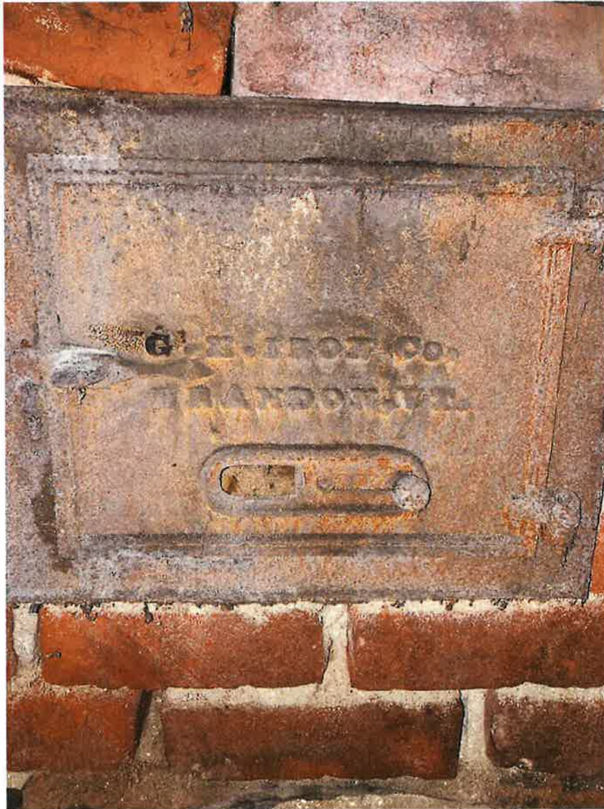
Pigeon House: Fire door of basement stove
