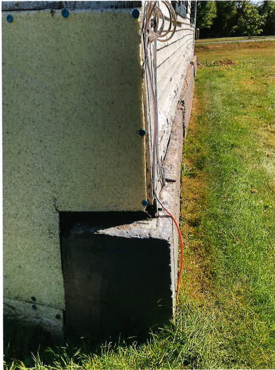
Pigeon House, Westford, Vt. NE corner at rear with deteriorating trim and siding
