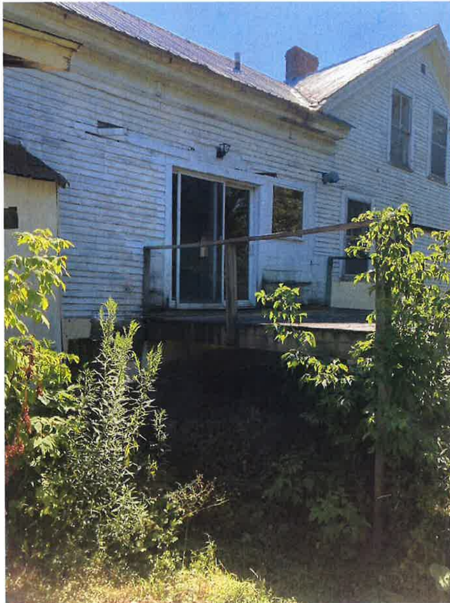
Pigeon House, Westford, Vt. Rear wall with failing deck and failed basement wall.
