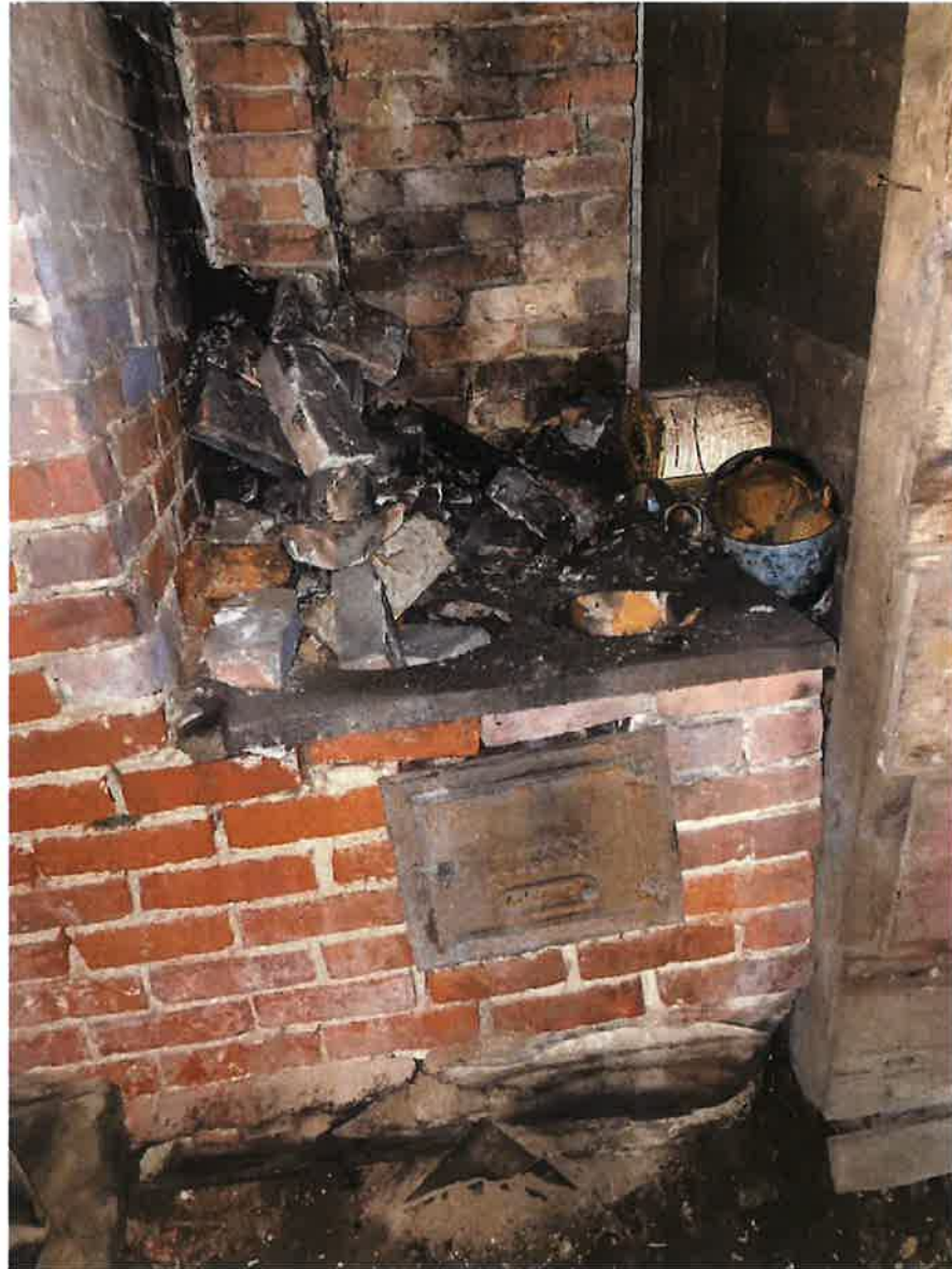
Pigeon House: Brick with cast iron cook surface and fire door adjacent to the bake oven in basement
