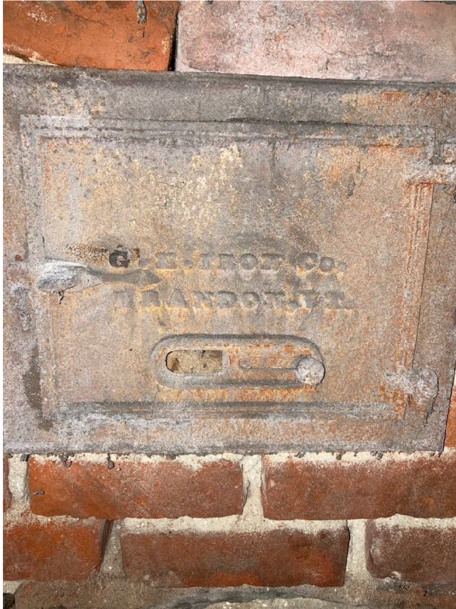
Pigeon House: Fire door of basement stove
