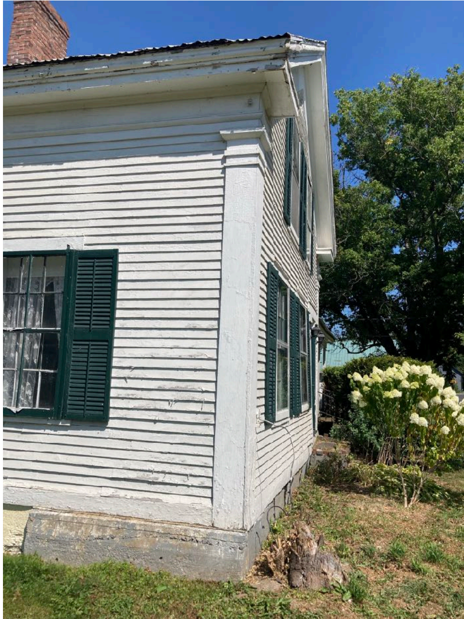
Pigeon House, NW corner with front wall slightly bowed
