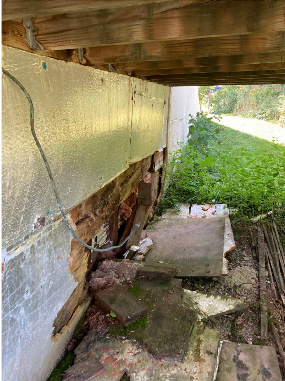
Pigeon House: failed rear wooden basement wall
